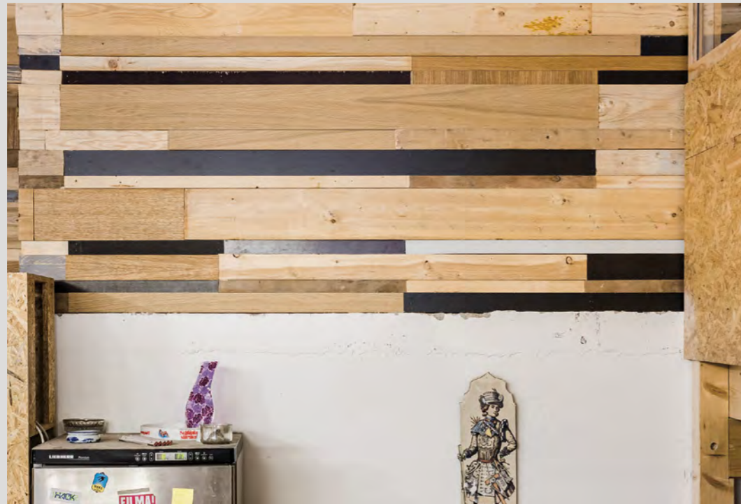
FIG. 14 Scraps of wood in various shapes and colors were reused as wall paneling in the Rollwerk workshop's kitchen.
